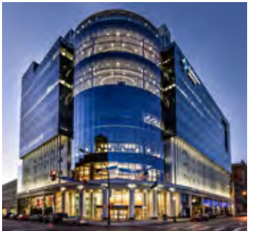
The Delaware North Building in Buffalo, N.Y., receives a statewide award for Excellence in Mixed-Use Development from the Urban Land Institute (April 3, 2017)
